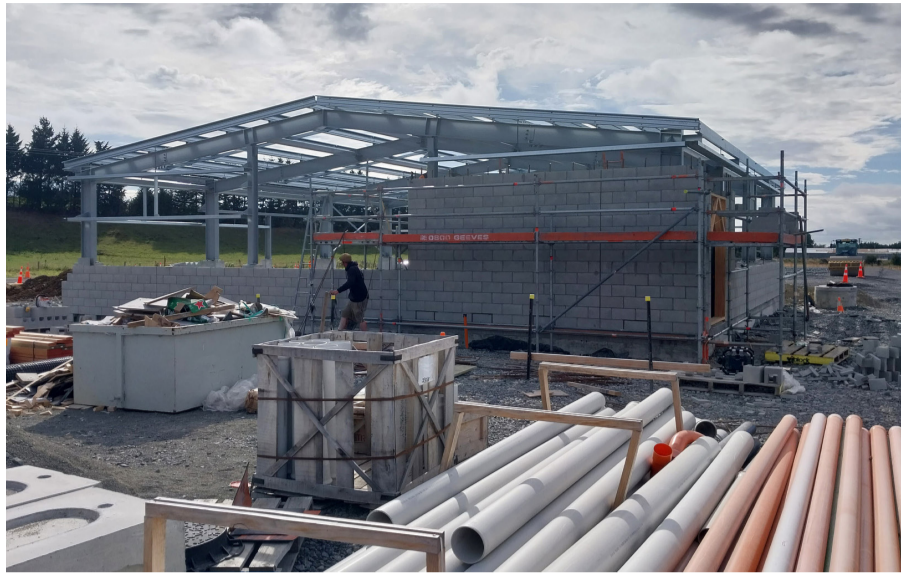
The new Mount Somers water treatment plant under construction.
