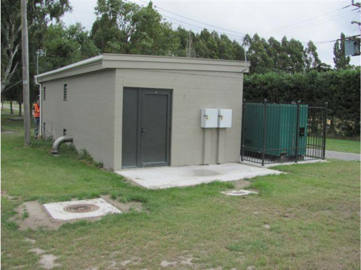
Photo 1: Water treatment plant and generator
