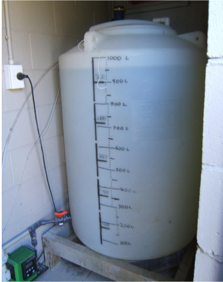
Photo 5: Sodium hypochlorite storage tank and pump
