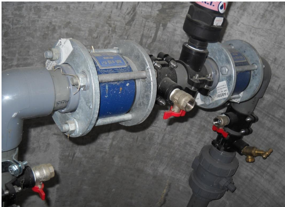
Inside of Borehead Chamber
