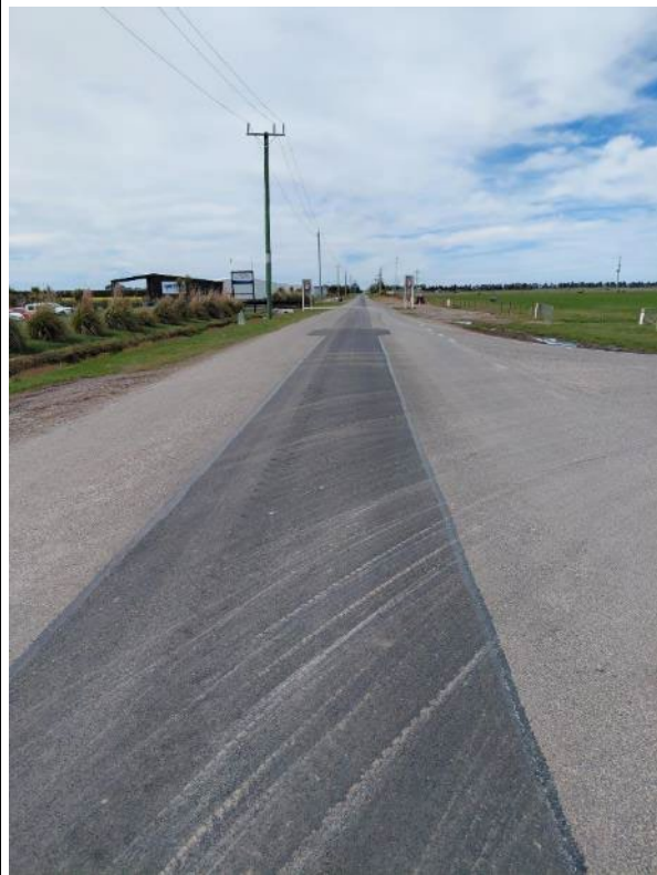
Line Road Sewermain Renewal (Trueline Civil Limited)
