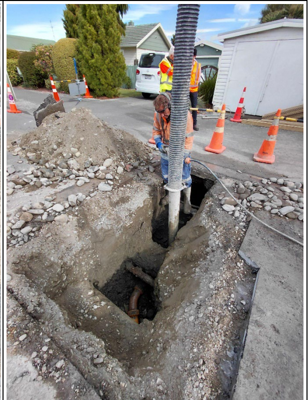
Bridge Street Sewer Lateral Repair (Ashburton Contracting Limited)
