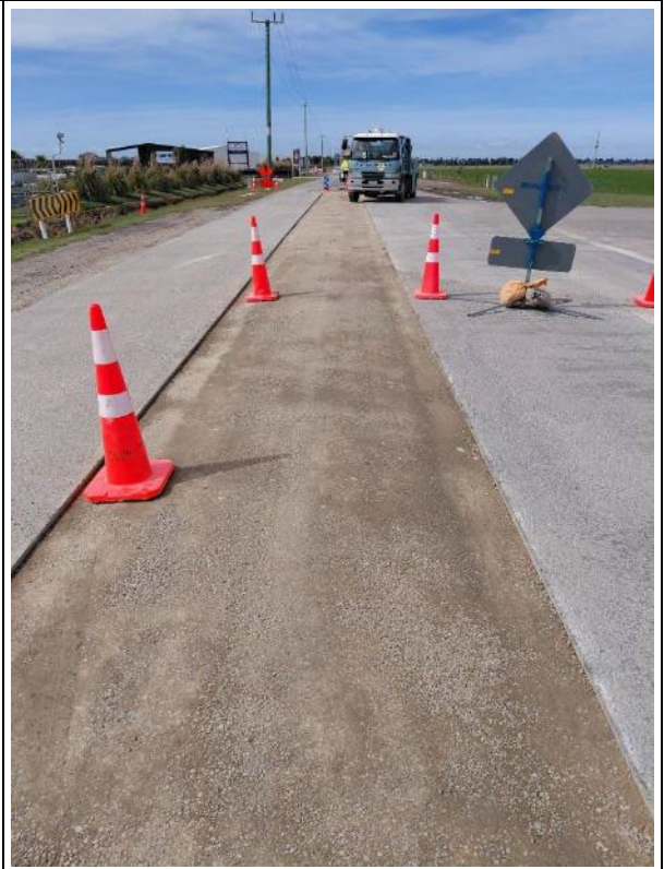
Line Road Sewermain Renewal (Trueline Civil Limited)
