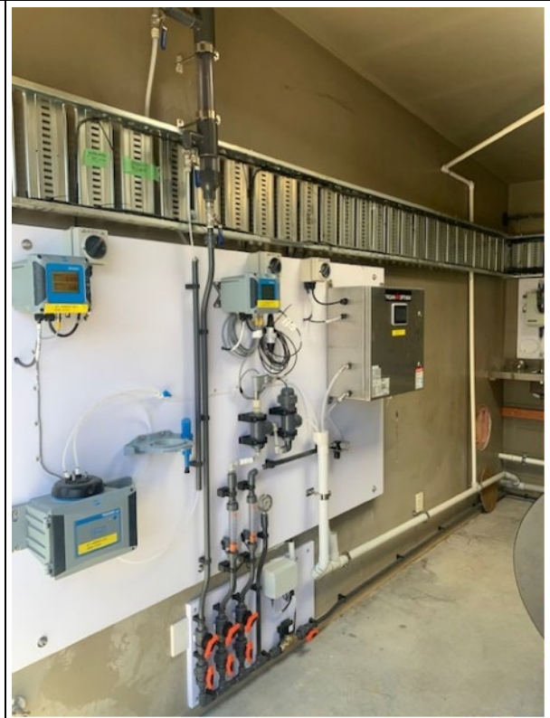
Bridge Street WTP UV Upgrade (ARC Projects Limited)
