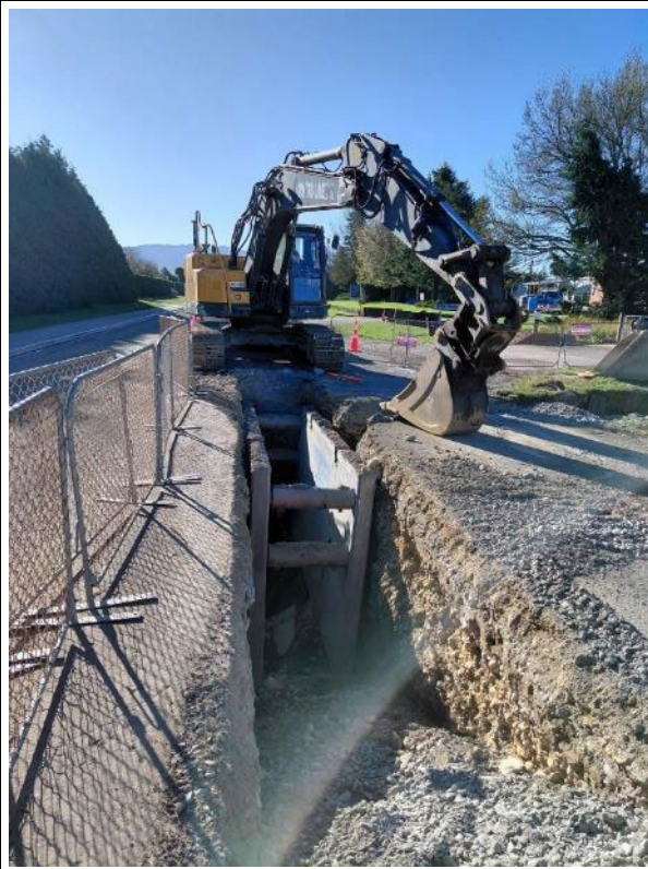
Line Road Sewermain Renewal (Trueline Civil Limited)
