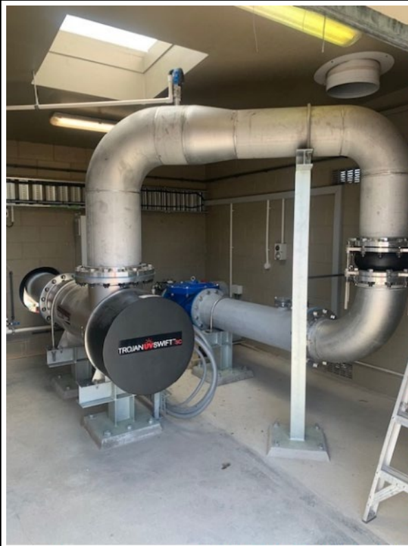
Bridge Street WTP UV Upgrade (ARC Projects Limited)
