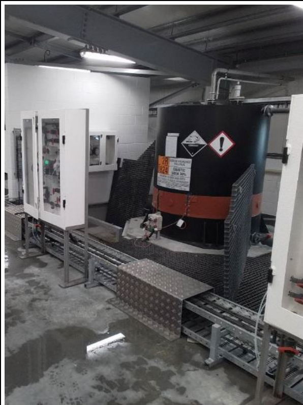
Methven WTP Caustic Soda Pump Repair (Ashburton Contracting Limited)
