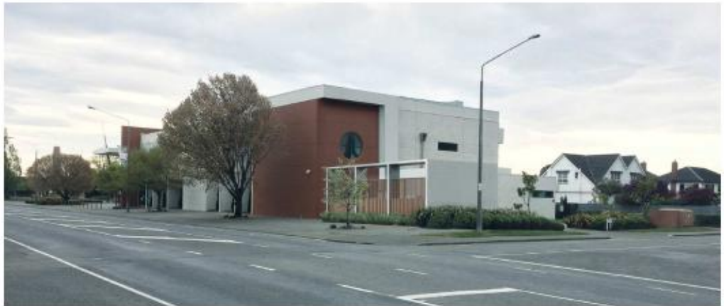
Plant enclosure looking west from SH1
