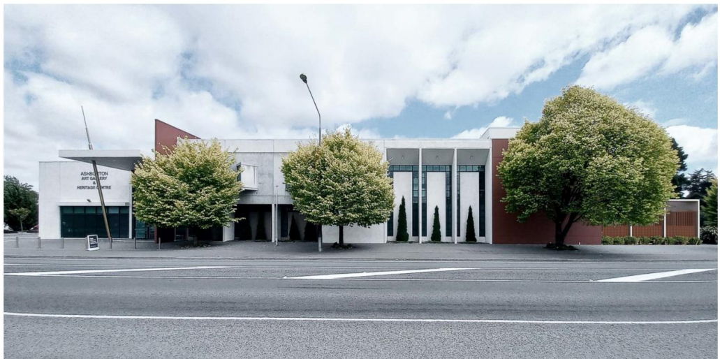
Plant enclosure looking north-west from SH1.
