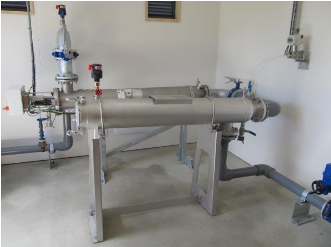
Photo 7: UV and filtration units
