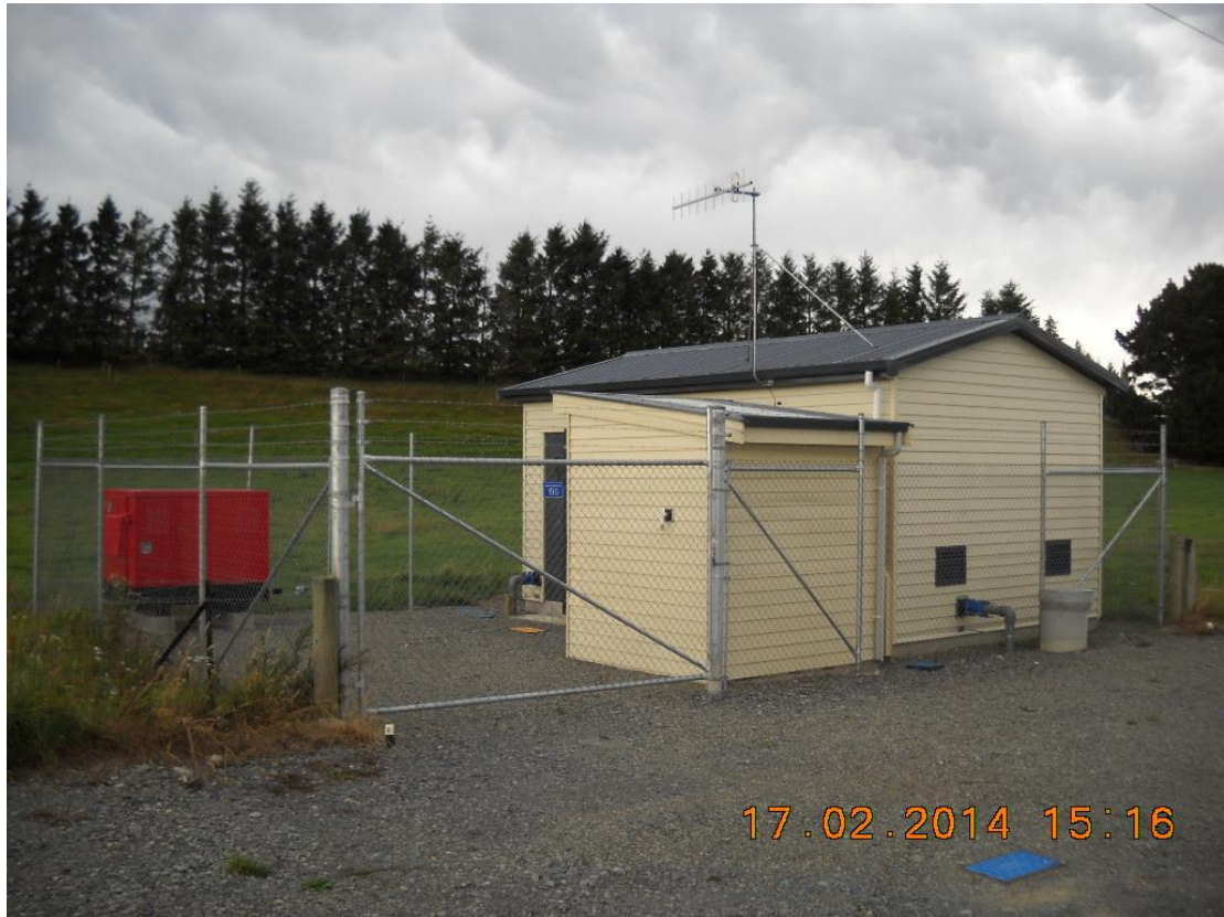
Photo 3: Treatment plant and generator
