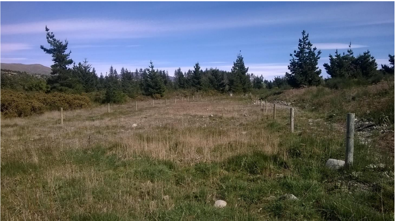
Photo 2: Intake gallery fenced compound with far manhole in the distance
