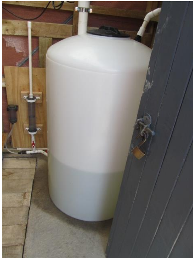
Photo 10: Chlorine tank
