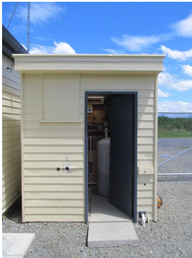
Photo 4: Chlorine dosing shed
