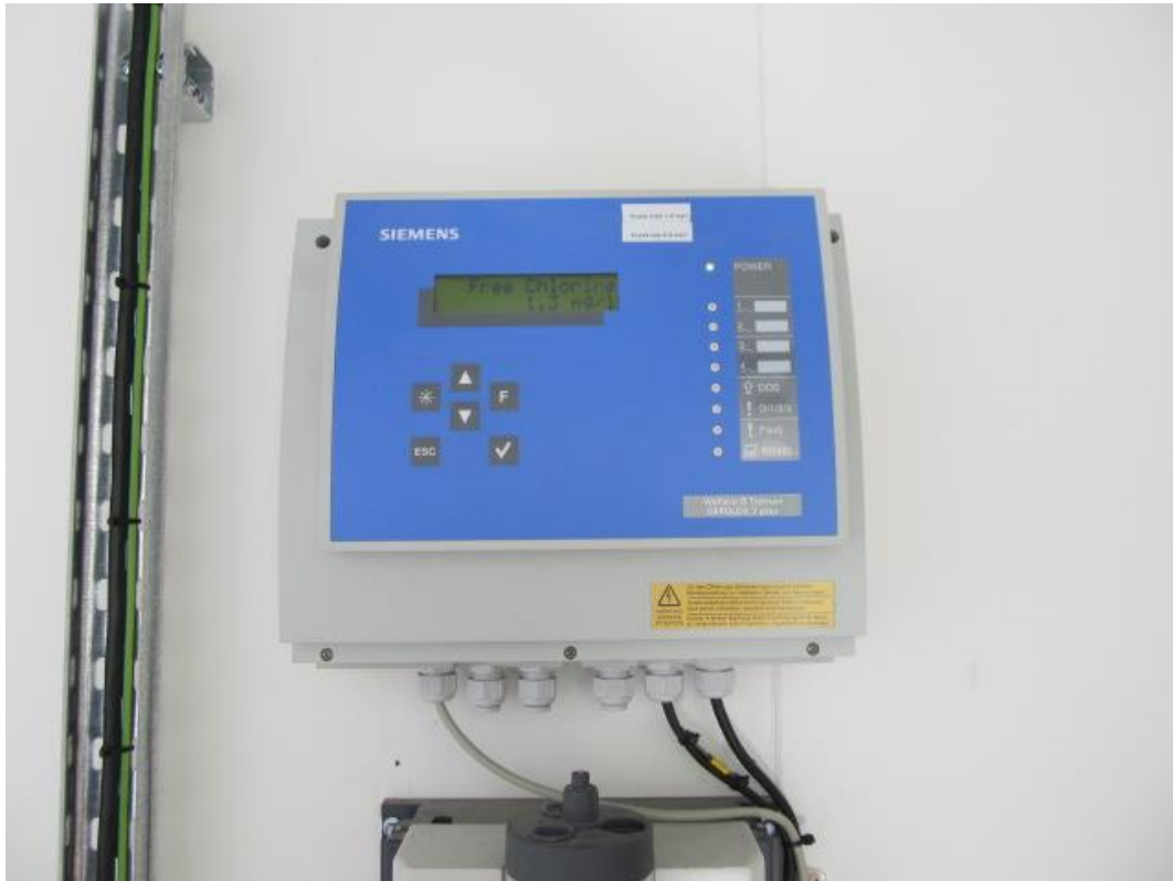
Photo 11: Chlorine analyser
