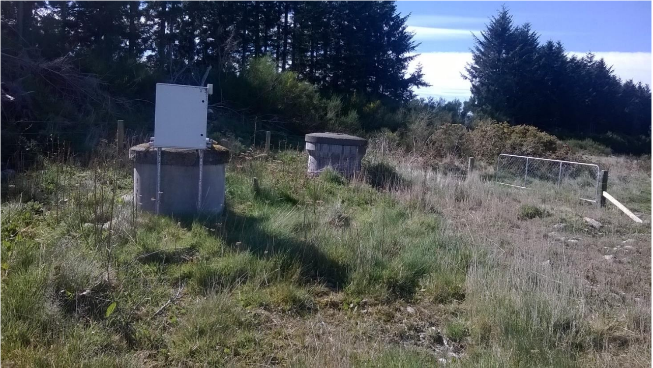
Photo 1: Intake gallery manholes inside locked compound
