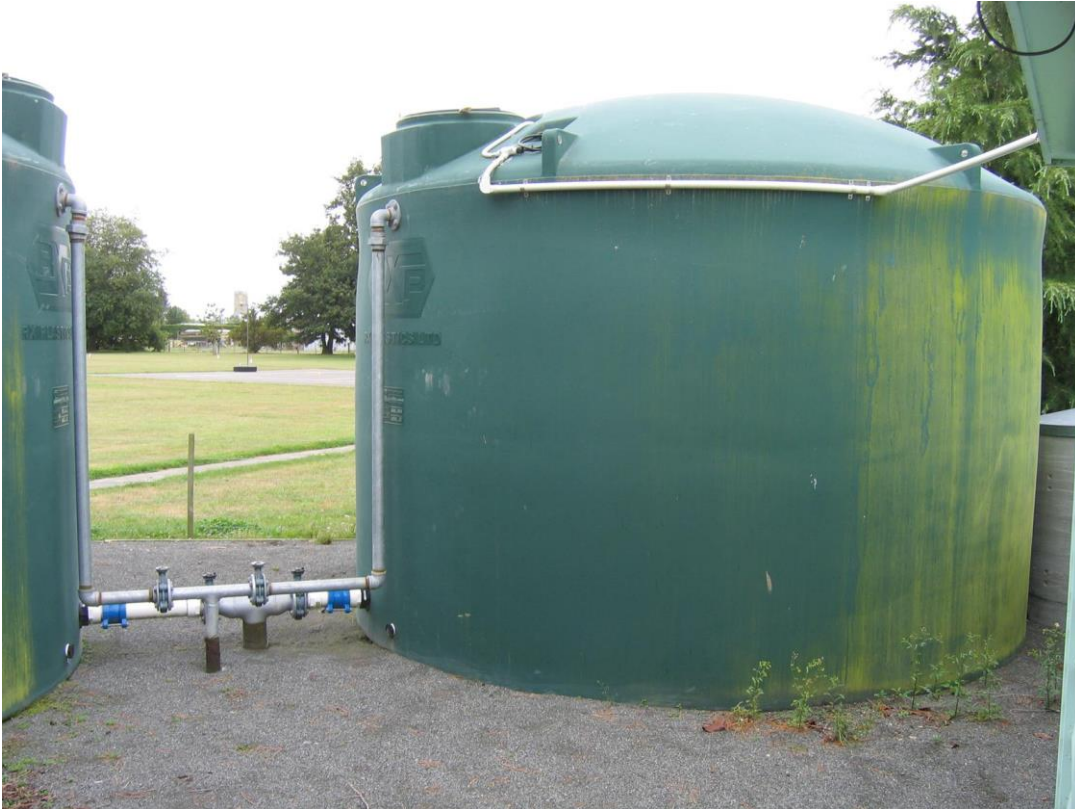
Figure 7 - Two 30m 3 Supply Reservoirs
