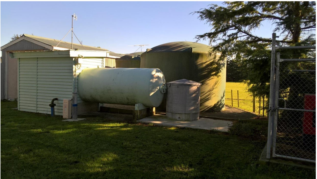
Figure 13: Chertsey Water Treatment Plant
