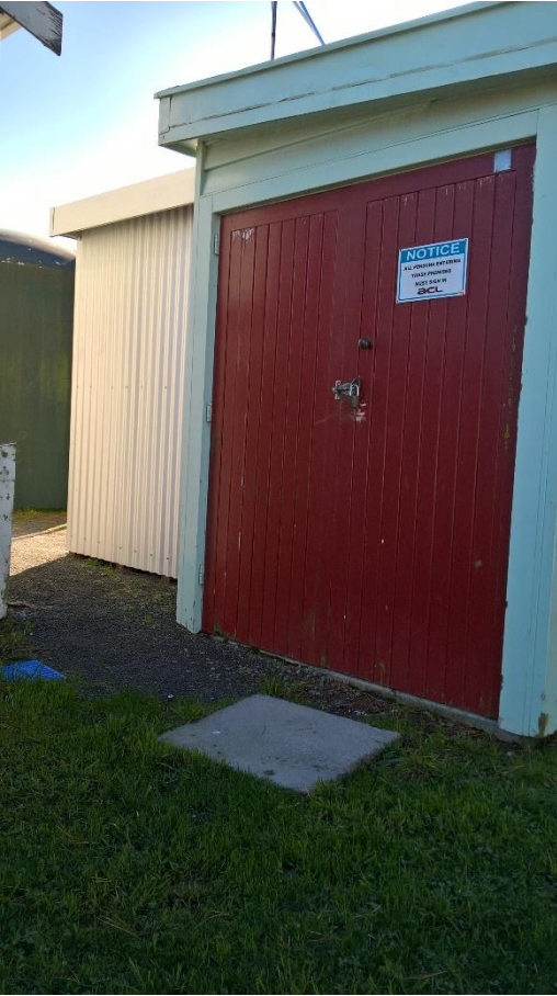
Figure 9 – Chertsey Pump Station Shed
