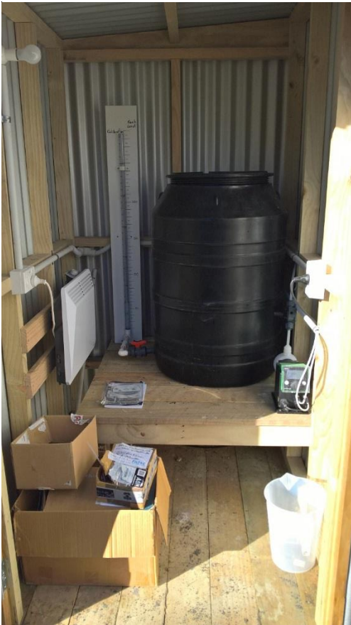
Figure 12: Chlorine Dosing Facility
