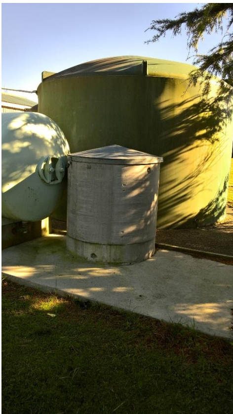
Figure 6 - Outside of Bore Enclosure
