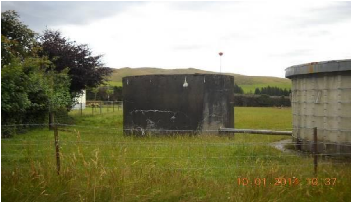
Figure 13 – Smaller reservoir connected to larger 70000L Reservoir on Chapmans Road
