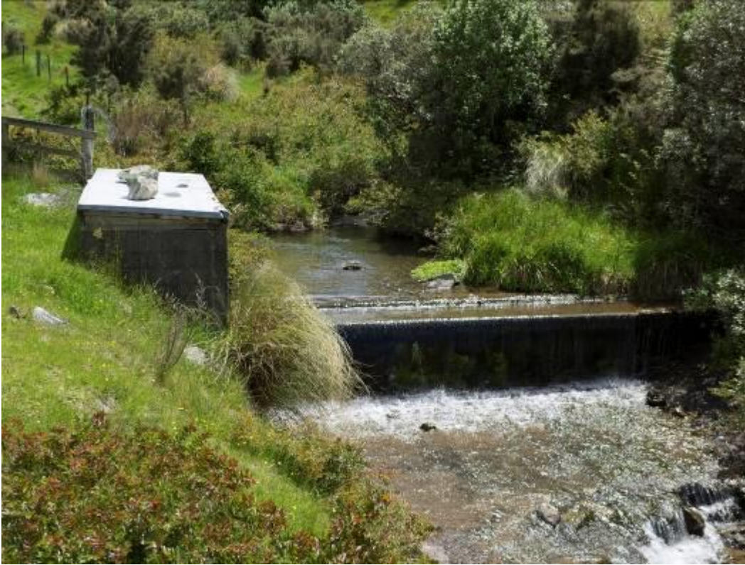
Figure 4 - Intake structure on the Hinds River, south branch - Weir A
