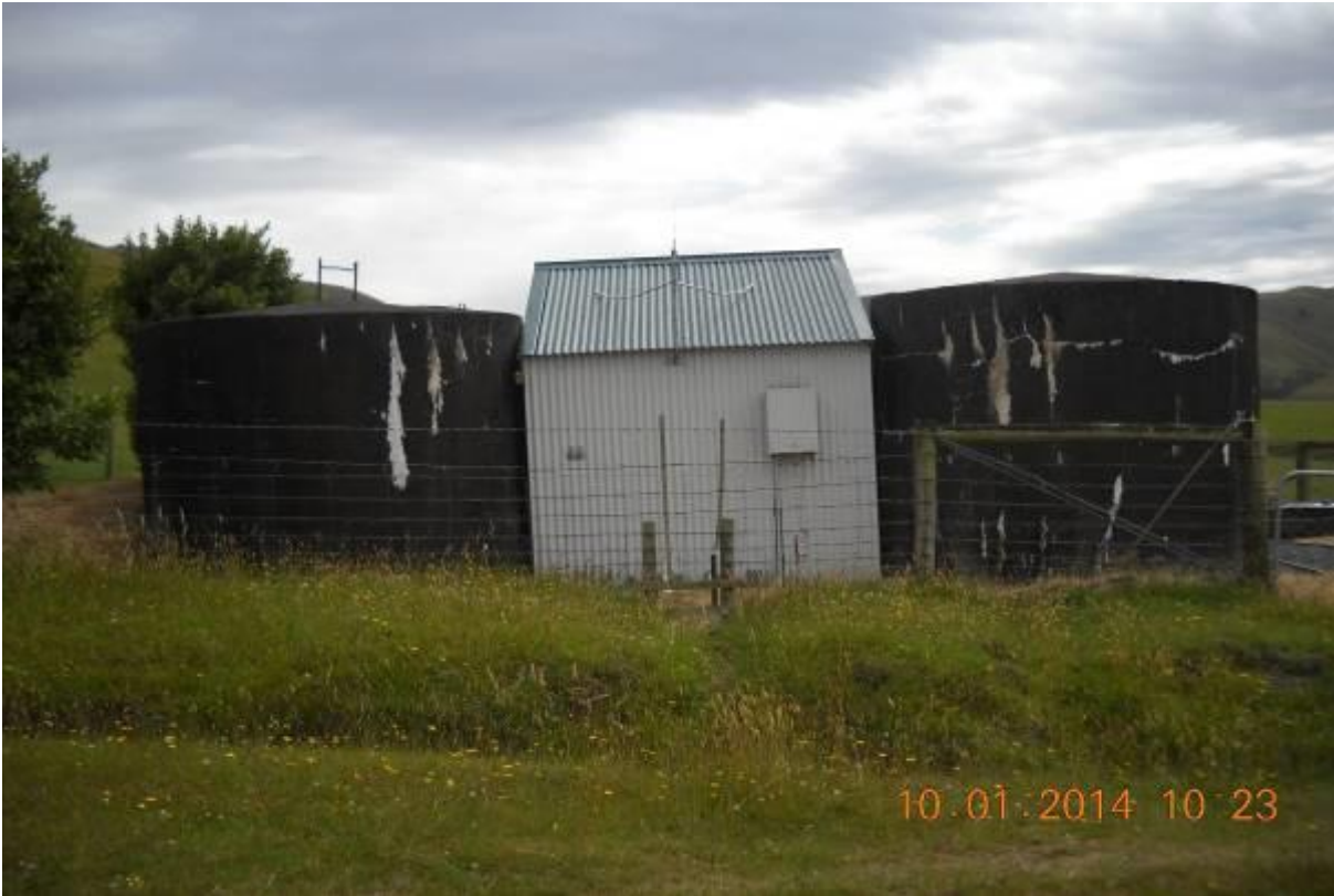
Figure 9 - Treatment shed and storage reservoirs
