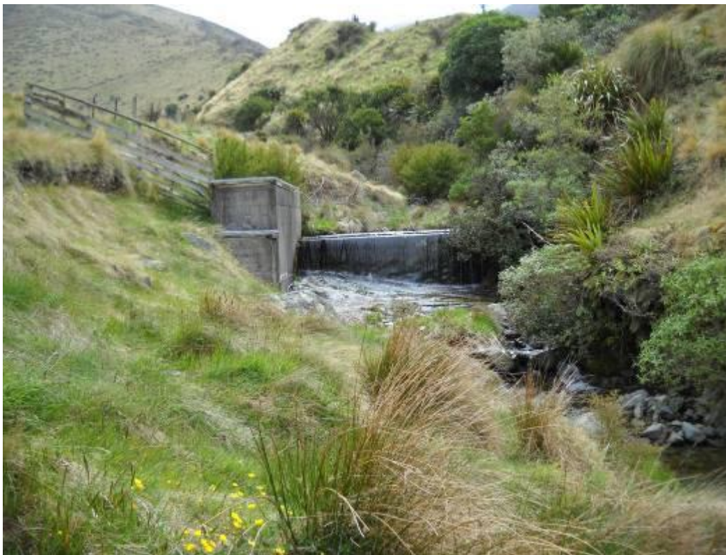
Figure 5 - Intake structure on the unnamed tributary - Weir B
