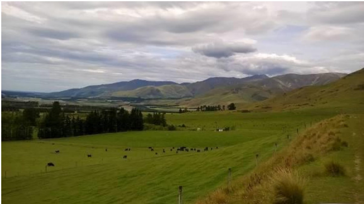
Figure 8 – Raw water trunkmain route (looking from intake access track to treatment plant)
