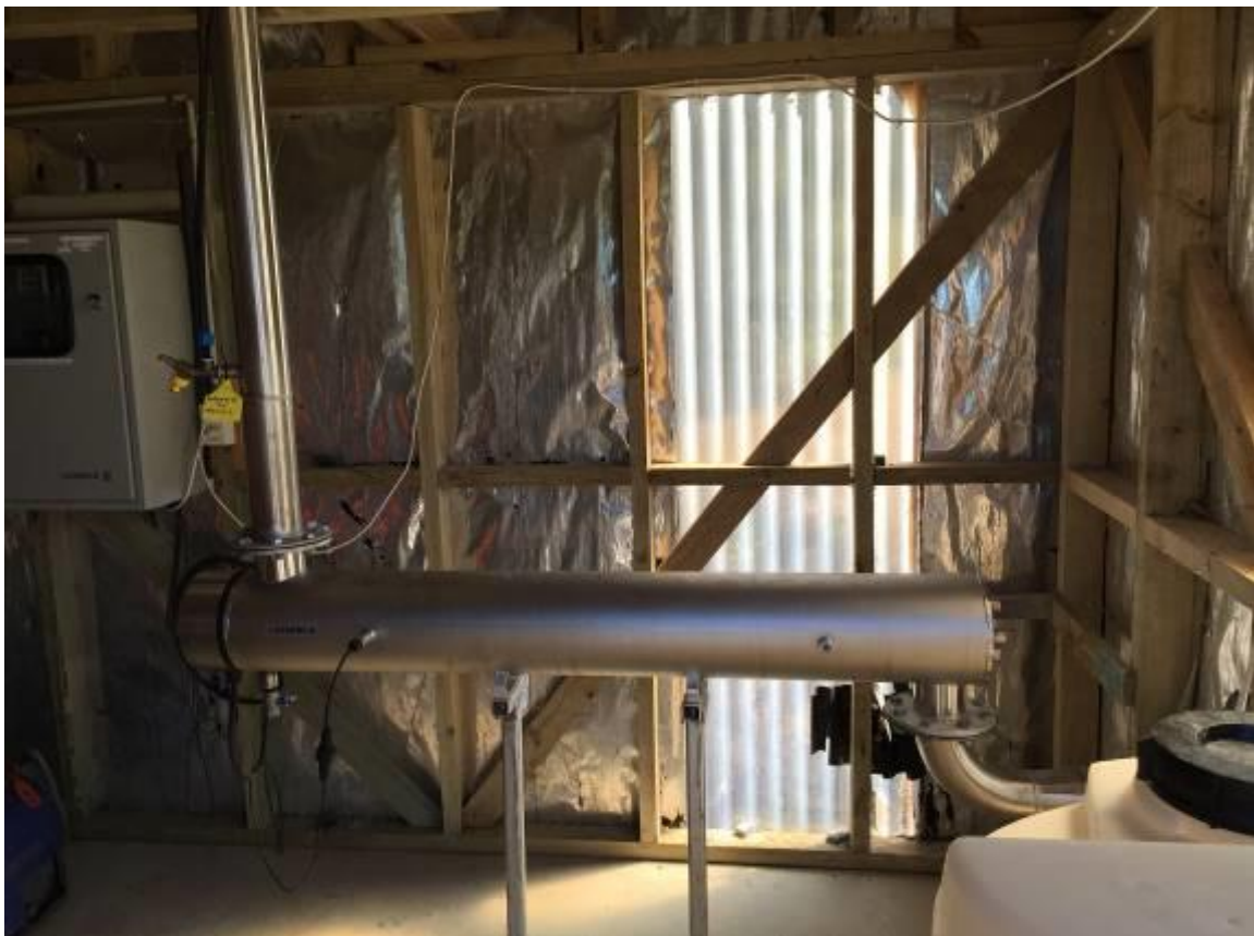
Figure 10 - UV unit within treatment plant
