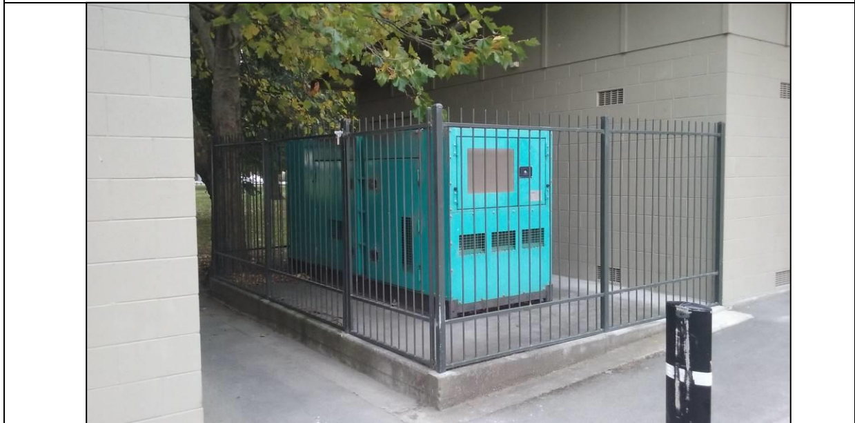
Figure 9: Argyle Park Generator
