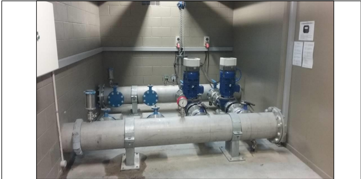
Figure 8: Argyle Park Booster Pumps for Allenton Pressure Zone
