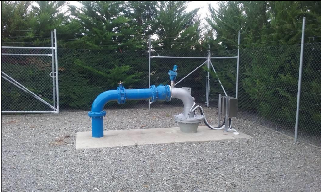
Figure 26: Tinwald Bore Headworks
