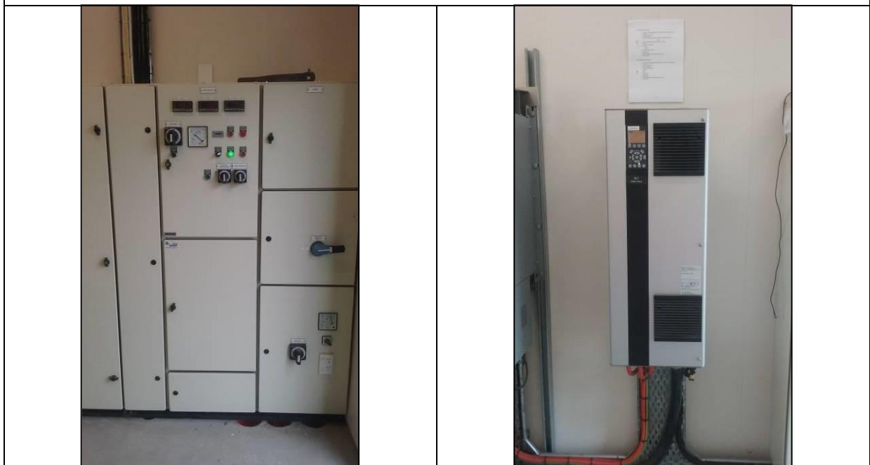
Figure 29: Tinwald Control Panel; Bore Pump Variable Speed Drive
