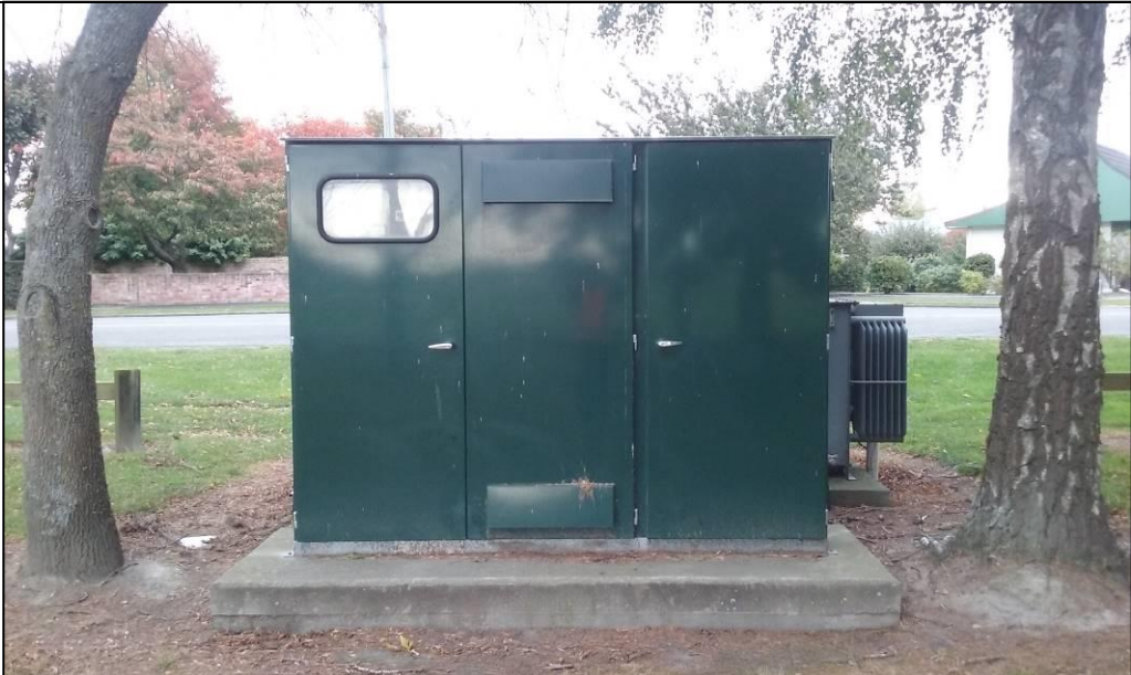
Figure 7: Argyle Park Bore 2 Control Unit (located separately from the main building)
