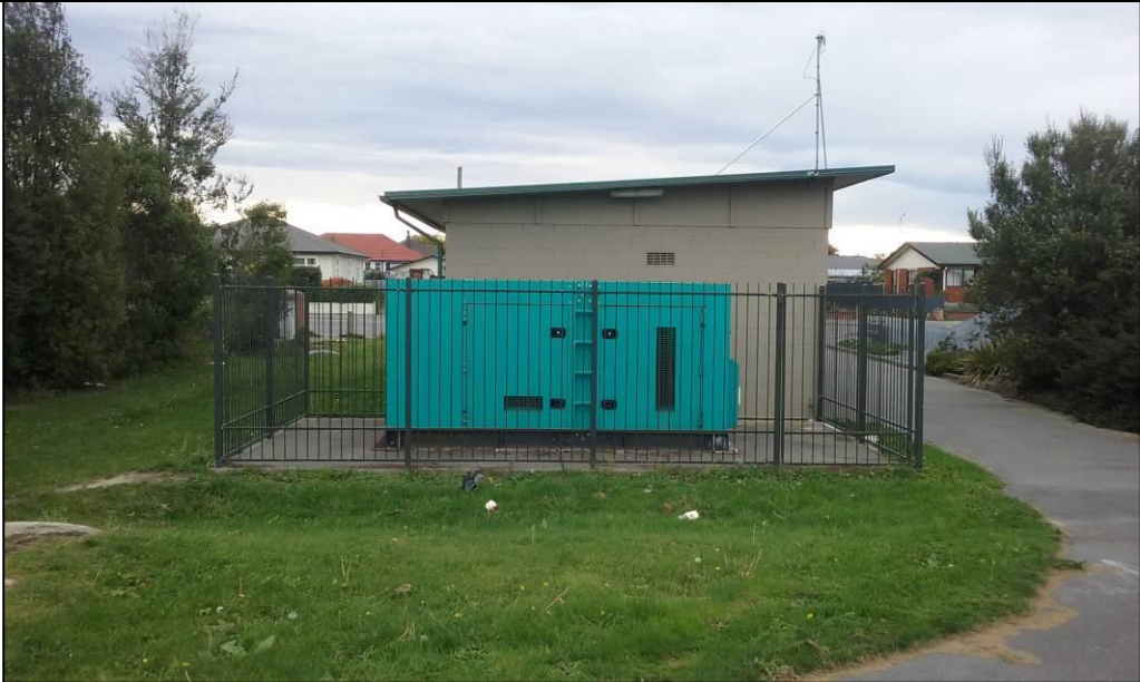
Figure 16: Bridge Street Generator
