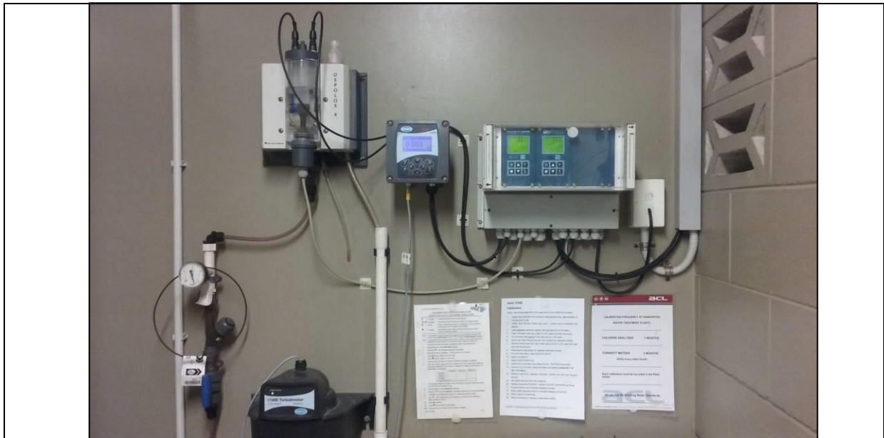
Figure 20: Domain Chlorine & pH Analyser
