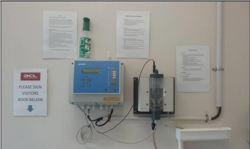
Figure 27: Tinwald Chlorine & pH Analyser
