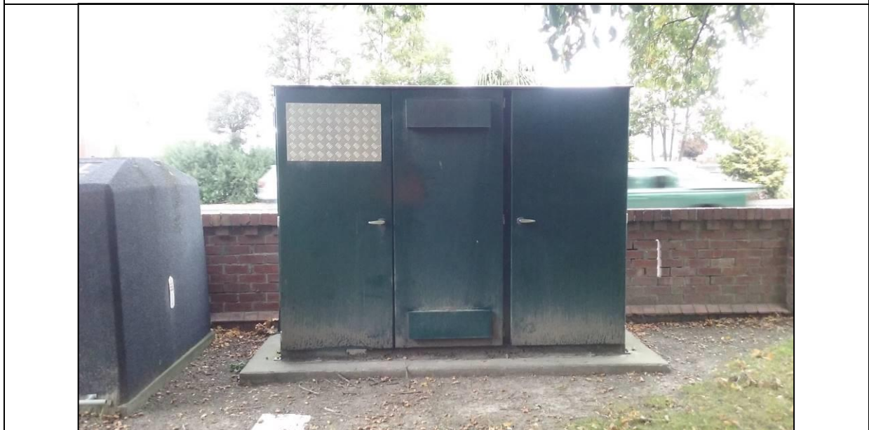
Figure 23: Domain 5 Control Unit (located separately from the main building)
