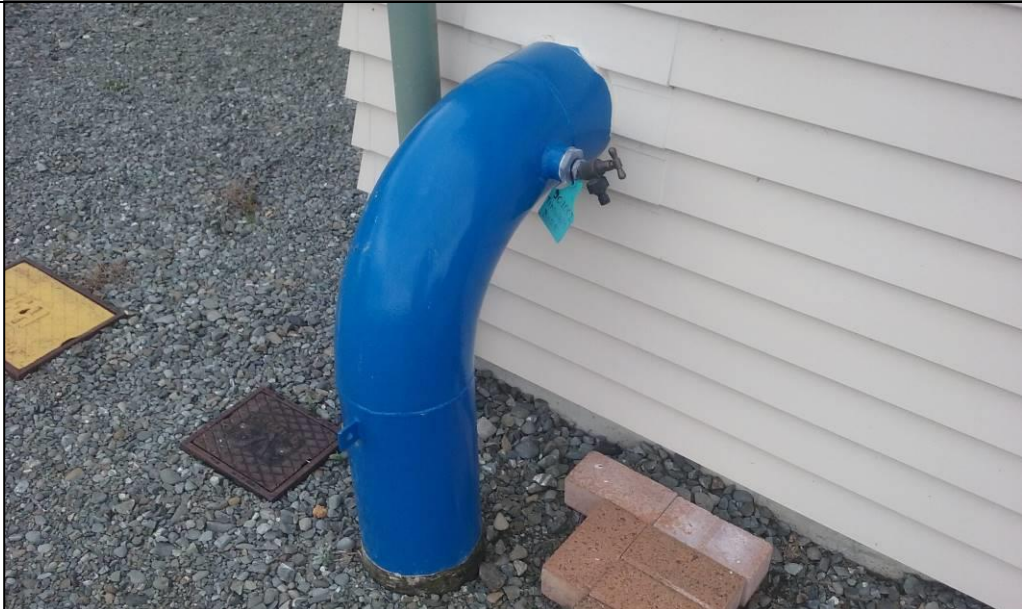
Figure 25: Tinwald Bore Sample Bollard
