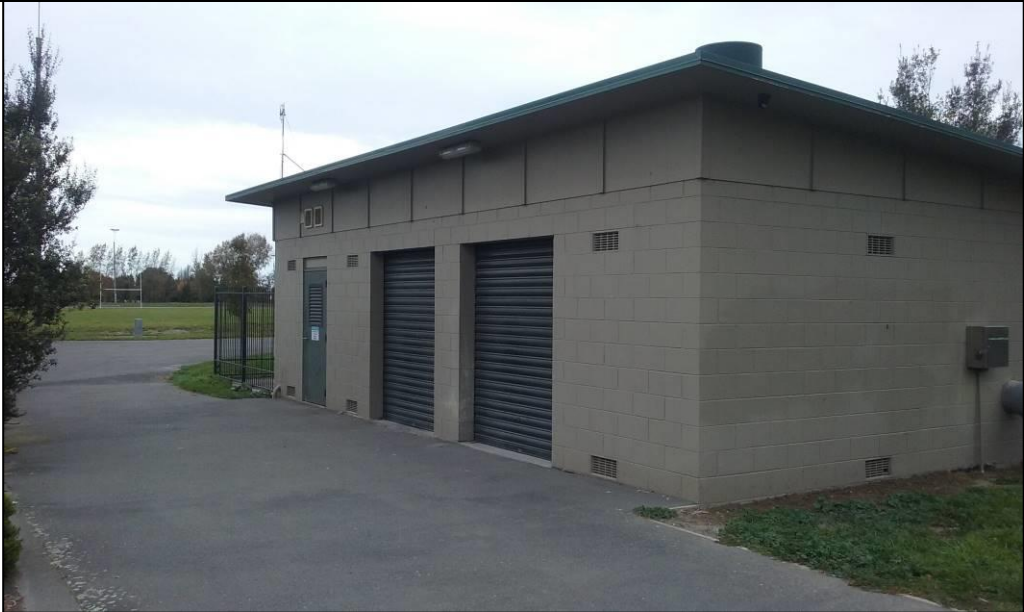
Figure 10: Bridge Street Treatment Building
