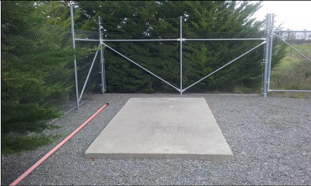
Figure 30: Tinwald Generator Pad (see improvements section for generator comments)
