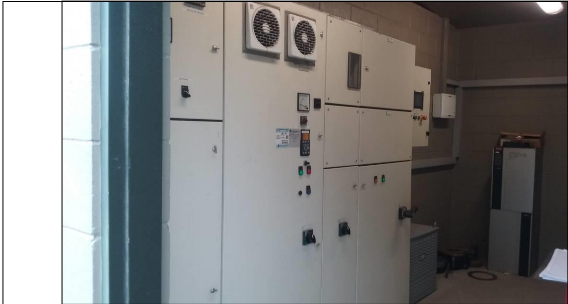
Figure 14: Bridge Street Bore 1 Control Panel (inside main treatment building)
