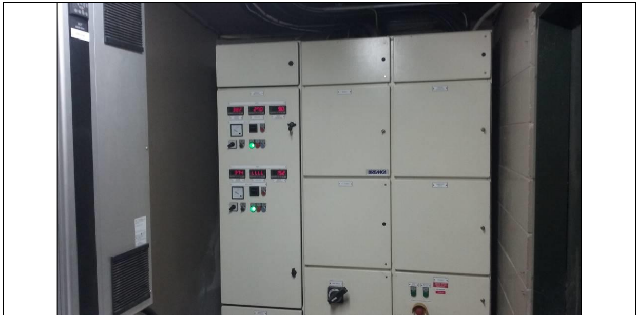
Figure 22: Domain Control Panel (inside main treatment building)
