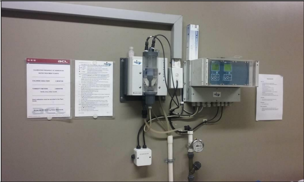
Figure 12: Bridge Street Chlorine & pH Analyser
