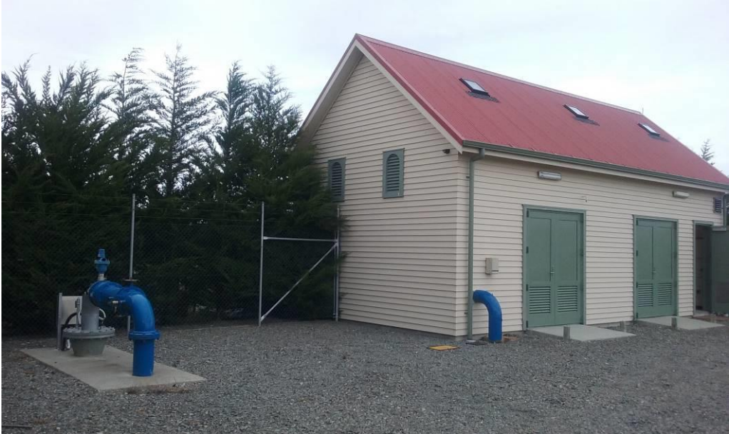
Figure 24: Tinwald Treatment Building and bore headworks
