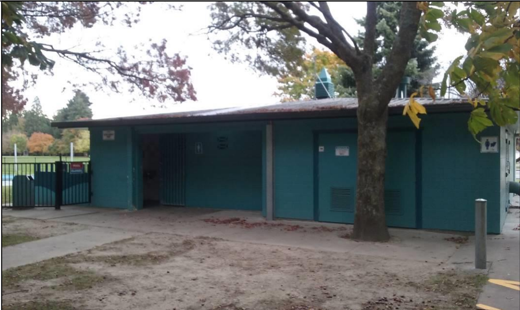
Figure 17: Domain Treatment Building
