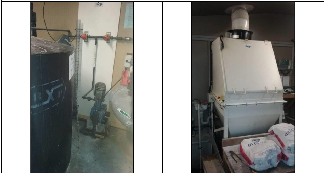
Figure 21: Domain Chlorine dosing pump and equipment; lime hopper
