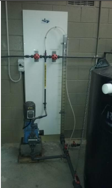
Figure 5: Argyle Park Chlorine dosing pump and equipment; lime hopper
