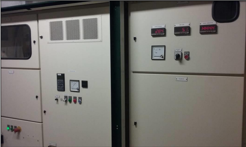
Figure 6: Argyle Park Bore 1 Control Panel (inside main treatment building)
