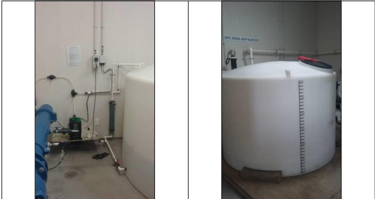
Figure 28: Tinwald Chlorine dosing pump and equipment; soda ash tank
