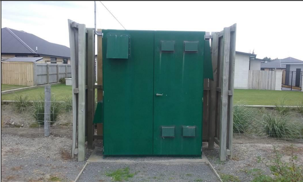
Figure 15: Bridge Street Bore 2 Control Unit (located separately from the main building)
