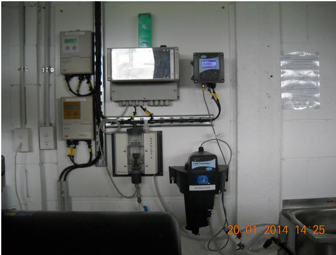
Photo 9: Flowmeter, chlorine and turbidity instrumentation
