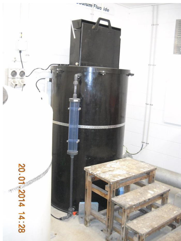
Photo 12: Fluoride dosing equipment
