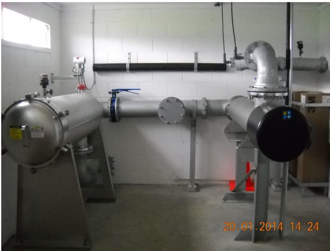
Photo 8: Cartridge filter (left) and UV unit (right)
