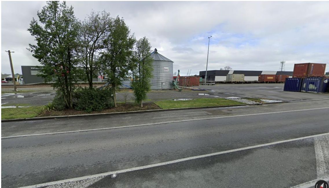
Figure 5: Southern end of site with adjoining railway land use (Source: Google Streetview)
