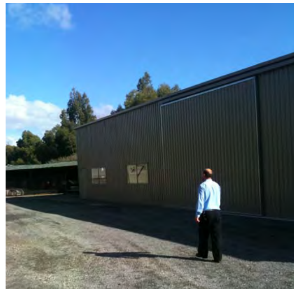
Steel profile and no overhang
