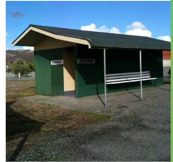
Concrete block walls and roof profile
