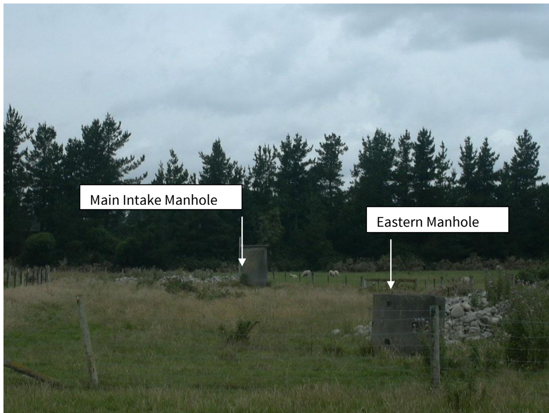
Photograph No 1 – Infiltration gallery, access chamber
