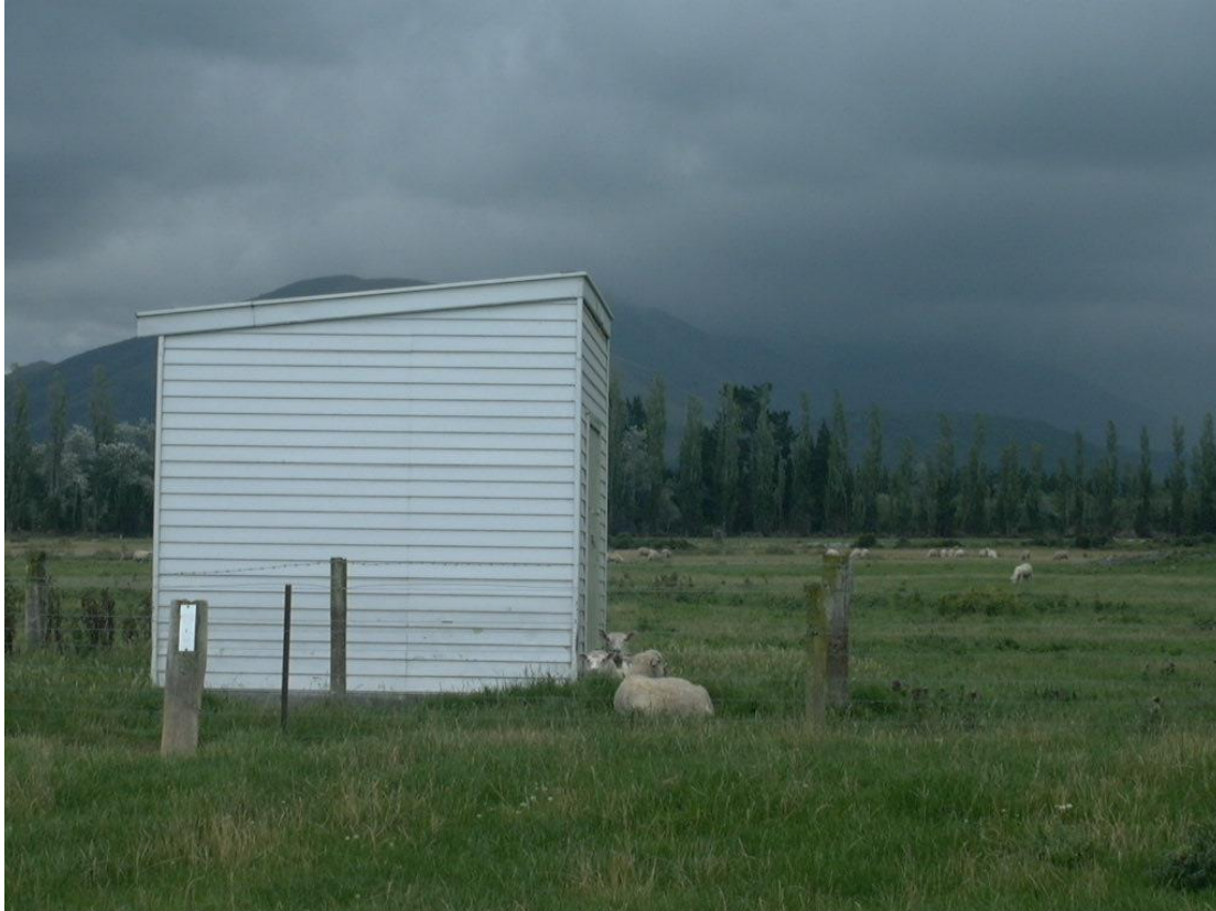
Photograph No 2 – Old chlorine shed on raw water trunkmain route
