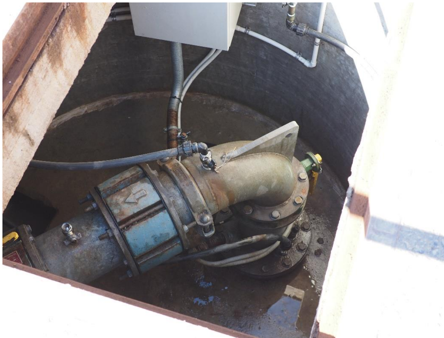
Inside of Borehead Chamber
