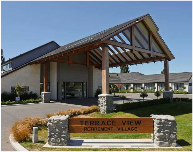
RIVERSTONE WALLS / COLUMNS TO MATCH EXISITNG RIVERSTONE USED WITHIN THE VILLAGE
