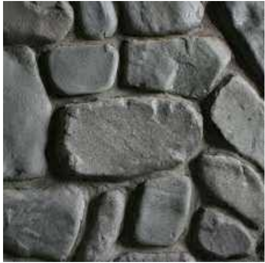
RIVERSTONE WALLS / COLUMNS TO MATCH EXISITNG RIVERSTONE USED WITHIN THE VILLAGE
