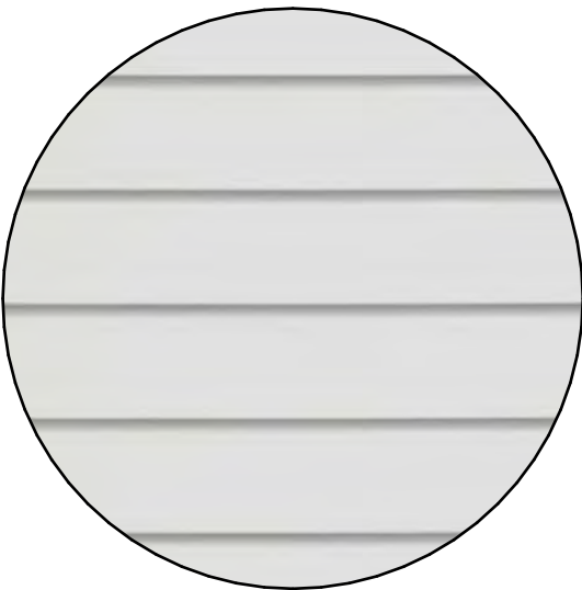
2. EXISTING WHITE TIMBER WEATHERBOARDS
