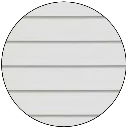
2. EXISTING WHITE TIMBER WEATHERBOARDS
