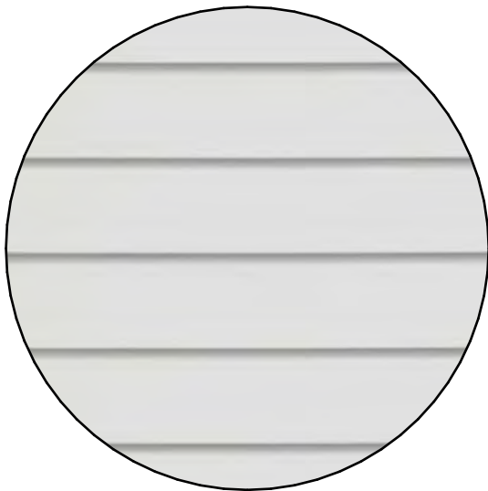
2. EXISTING WHITE TIMBER WEATHERBOARDS
