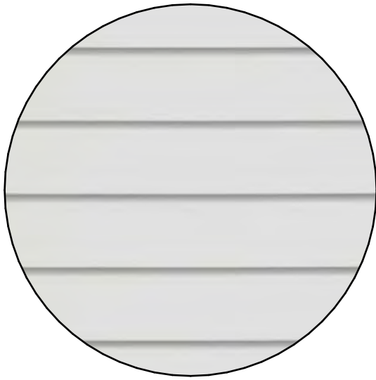
2. EXISTING WHITE TIMBER WEATHERBOARDS
