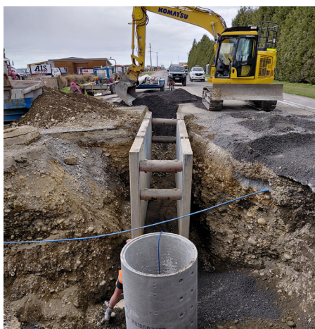
The new wastewater main on Line Road.
