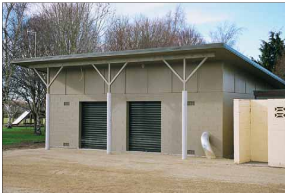
The new treatment plant at Argyle Park, which will treat water from two new deep bore wells at the park. There will be similar treatment facilities in the Ashburton Domain and Bridge Street from early next year.
