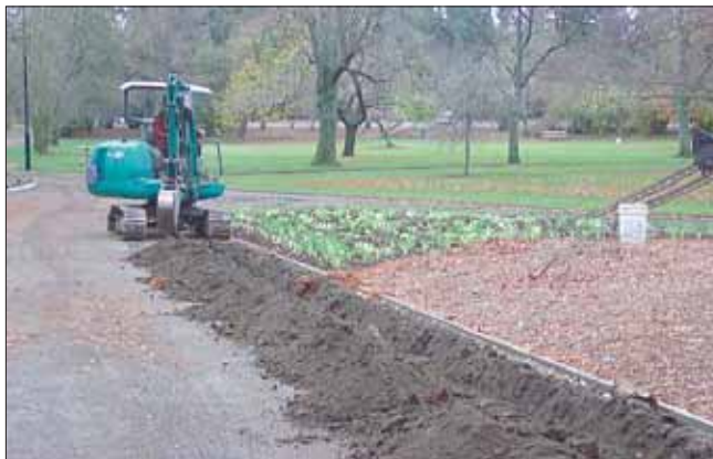
Digging irrigation trenches in the Ashburton Domain
